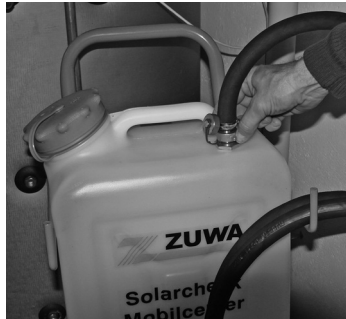
2. Connect return hose to the container.
